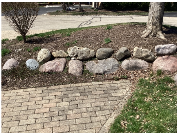
Stone retaining wall at the guest parking area
