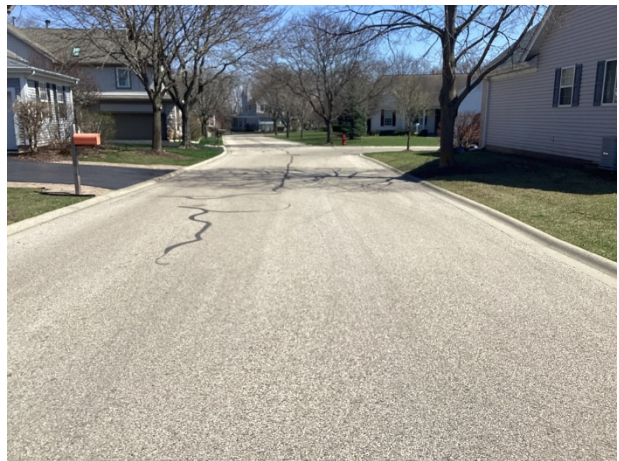
Norwich Court overview
