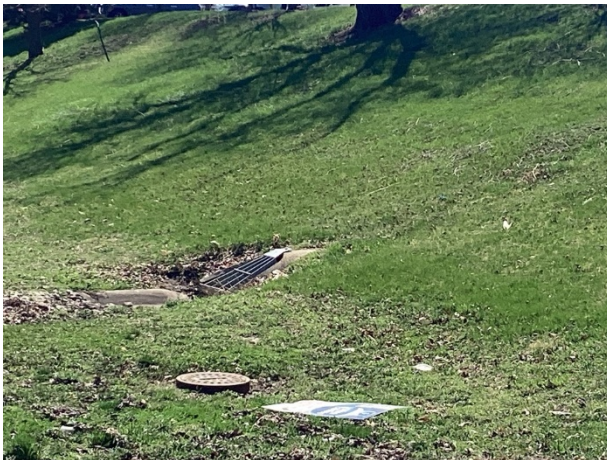
Small inlet structure
