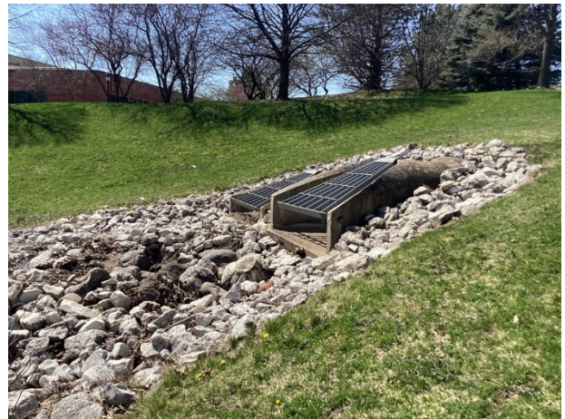
Main inlet structure
