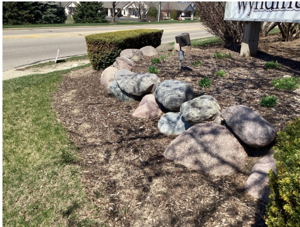
Stone retaining wall at the property entrance
