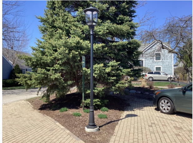
Recently installed light pole and fixture at Narragansett Court
