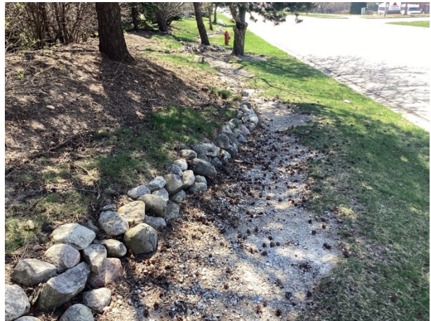
Stone retaining wall along the walking path
