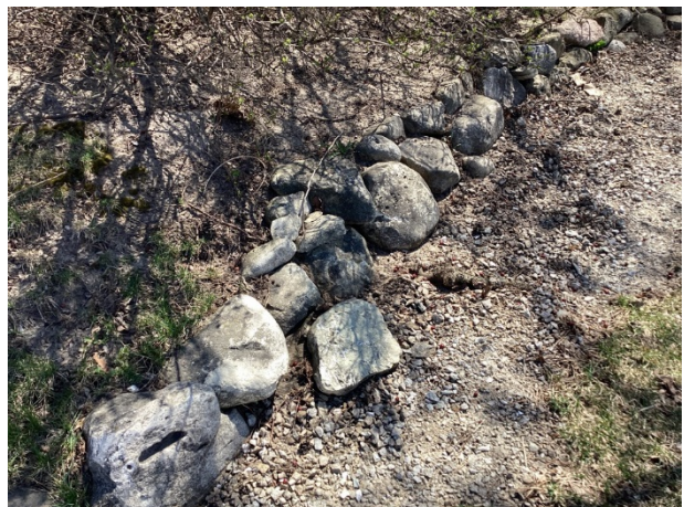
Loose stones along the walking path
