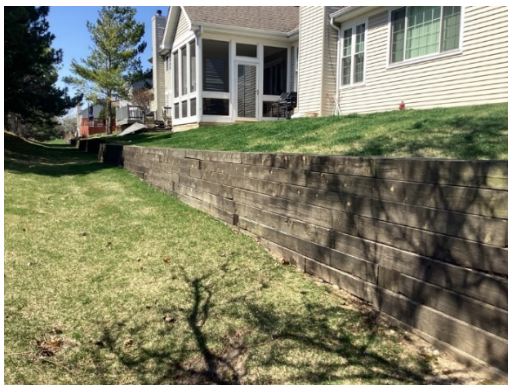
Retaining wall overview
