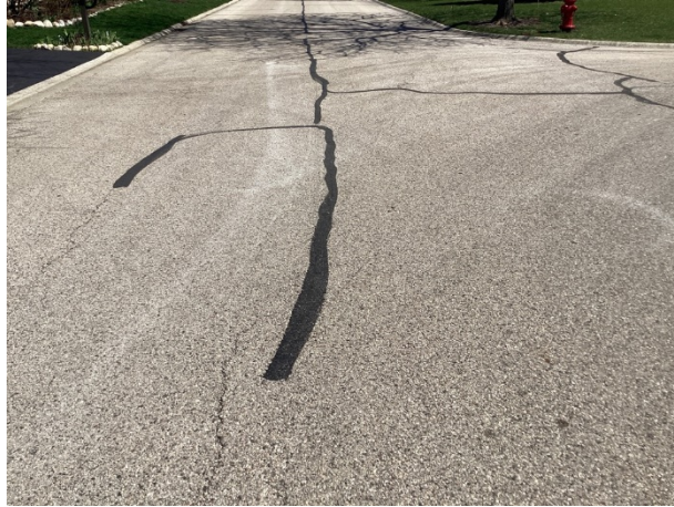
Recent crack repairs along center line of pavement at Norwich Court
