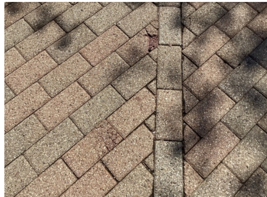
Damaged pavers
